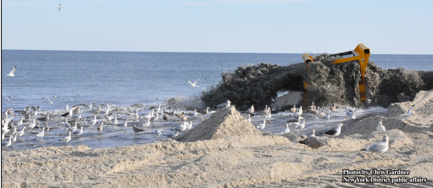
Army Corps personnel look for any unusual objects in a filter after sand is pumped onto the beach
