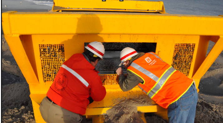
Army Corps personnel look for any unusual objects in a filter after sand is pumped onto the beach
